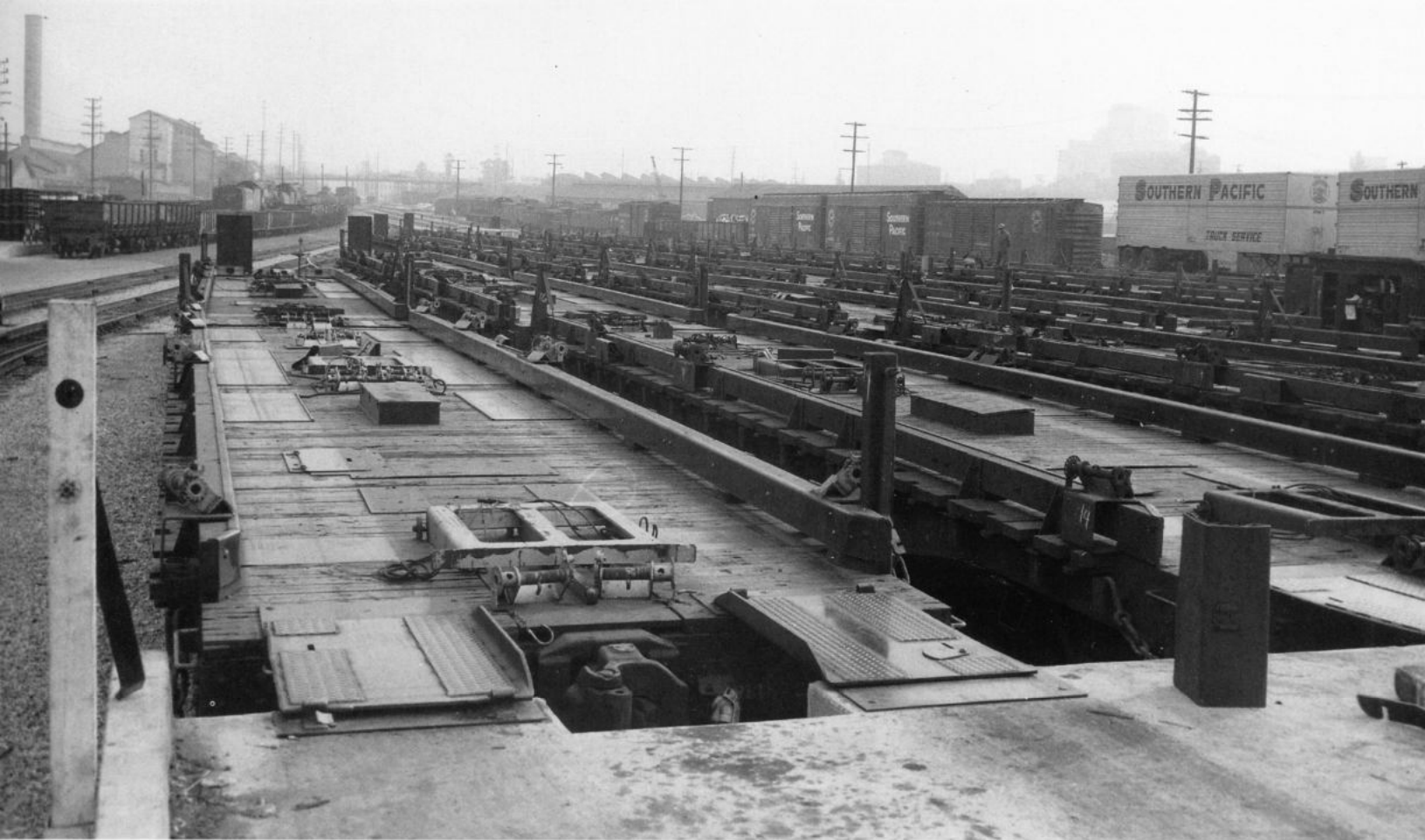
Operations soon outgrew the River Team Track at Los Angeles and a new six-ramp TOFC facility was opened during February 1955 adjacent the Alhambra Avenue Shops on the east side of the Los Angeles River. The Shops ramp, and the adjacent PMT facility, seen here in these early 1956 views, was the largest dedicated trailer-flatcar complex on the Pacific Lines and was expanded many times in succeeding years to encompass not only the entire area once occupied by the Alhambra Avenue roundhouse and Los Angeles Shops, but the adjacent Mission Road coach yard. —Three photos, Southern Pacific, John R. Signor collection
