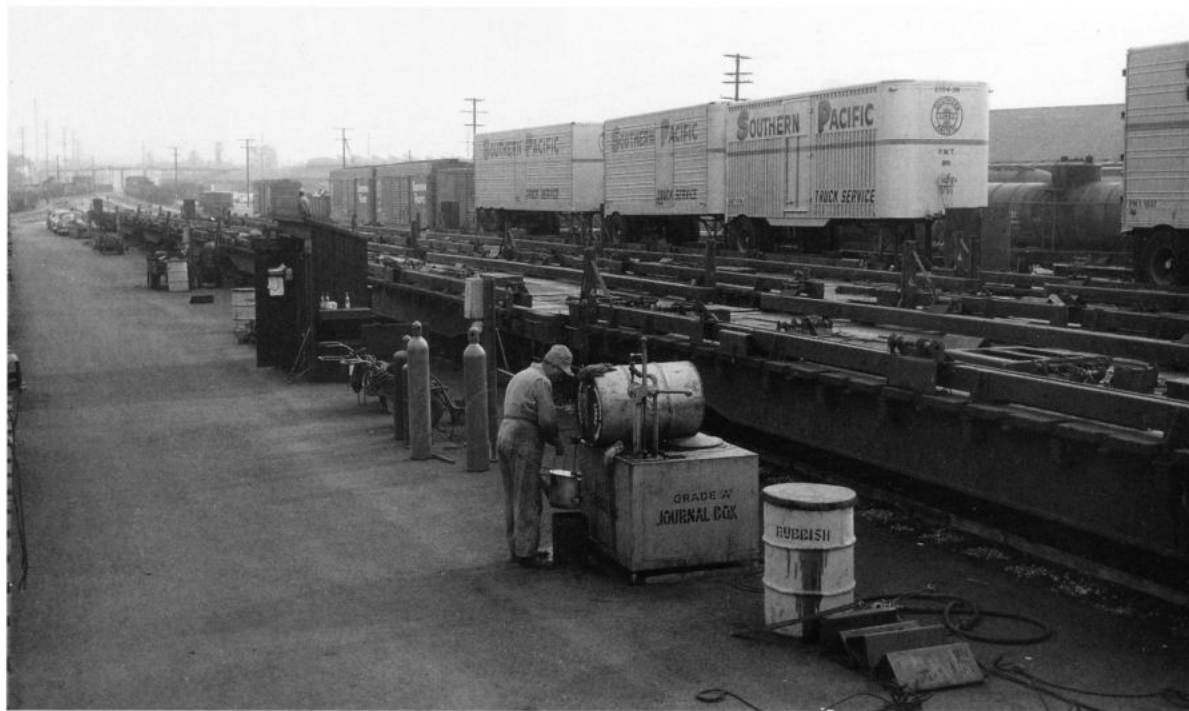
Operations soon outgrew the River Team Track at Los Angeles and a new six-ramp TOFC facility was opened during February 1955 adjacent the Alhambra Avenue Shops on the east side of the Los Angeles River. The Shops ramp, and the adjacent PMT facility, seen here in these early 1956 views, was the largest dedicated trailer-flatcar complex on the Pacific Lines and was expanded many times in succeeding years to encompass not only the entire area once occupied by the Alhambra Avenue roundhouse and Los Angeles Shops, but the adjacent Mission Road coach yard. —Three photos, Southern Pacific, John R. Signor collection
