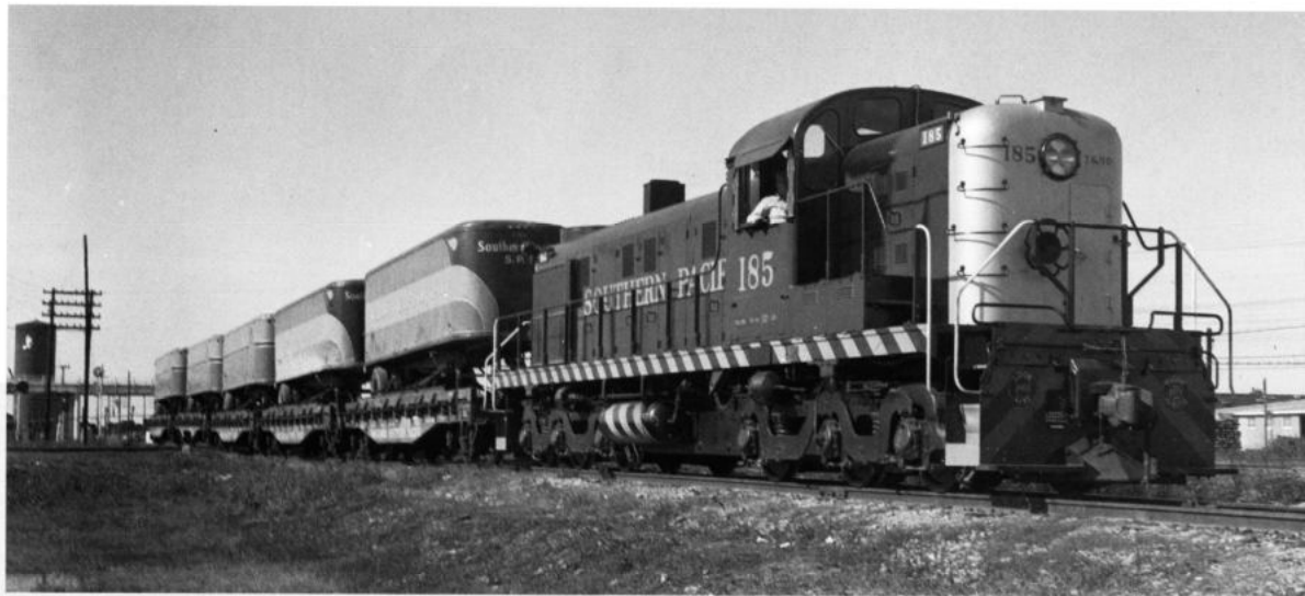
On this page and below opposite are early publicity views of T&NO's piggyback operations in the Houston area during the late spring of 1953. The trailers are a mix of Daylight -painted vans and earlier SPT equipment. Note security bars on the trailers in the lower view. —All, Southern Pacific, John R. Signor collection
