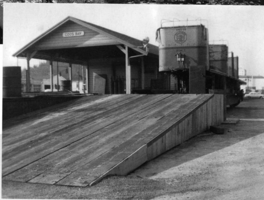
In the early years of TOFC service, SP just paved over an area near the railroad, added yard lights, a simple ramp and maybe an office of some sort. In these three views taken in early 1956, we see the piggyback facility at Brooklyn, above, Coos Bay, right, and Eugene, below. At one time or another other stations in Oregon with trailer-flatcar ramps included Albany, Klamath Falls, Medford, Salem, Roseburg and Tillamook. —All, Southern Pacific, John R. Signor collection
