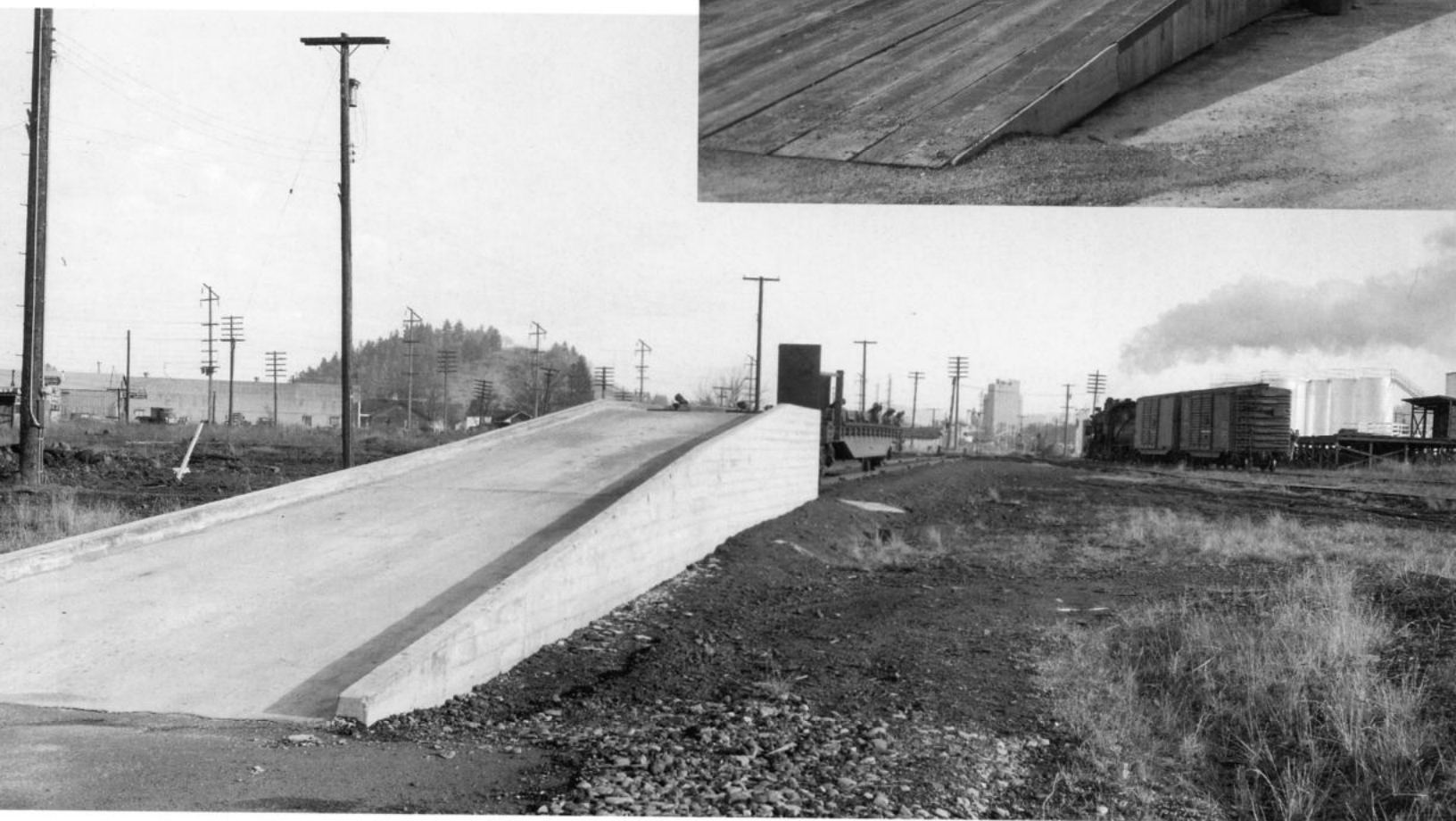
In the early years of TOFC service, SP just paved over an area near the railroad, added yard lights, a simple ramp and maybe an office of some sort. In these three views taken in early 1956, we see the piggyback facility at Brooklyn, above, Coos Bay, right, and Eugene, below. At one time or another other stations in Oregon with trailer-flatcar ramps included Albany, Klamath Falls, Medford, Salem, Roseburg and Tillamook. —All, Southern Pacific, John R. Signor collection
