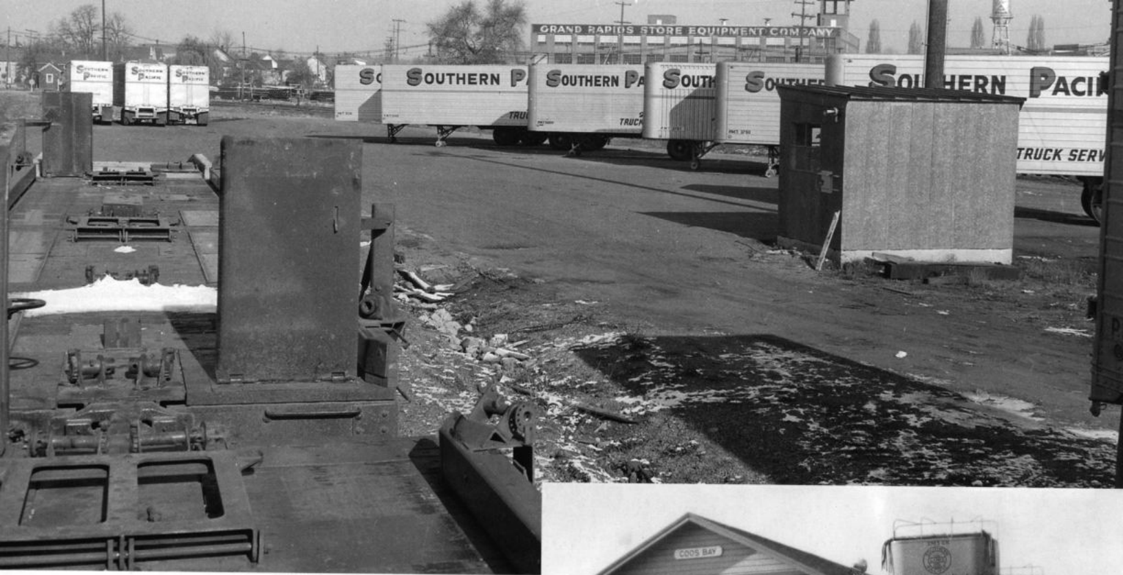
In the early years of TOFC service, SP just paved over an area near the railroad, added yard lights, a simple ramp and maybe an office of some sort. In these three views taken in early 1956, we see the piggyback facility at Brooklyn, above, Coos Bay, right, and Eugene, below. At one time or another other stations in Oregon with trailer-flatcar ramps included Albany, Klamath Falls, Medford, Salem, Roseburg and Tillamook. —All, Southern Pacific, John R. Signor collection
