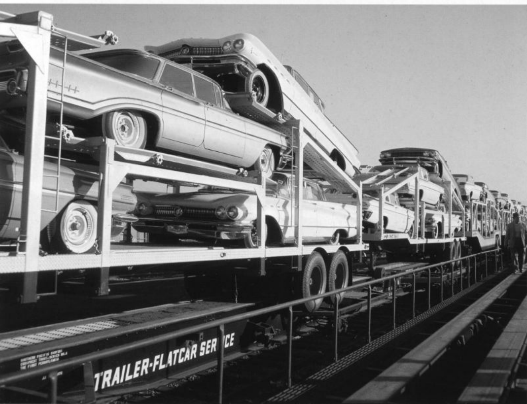
Train No. 336, the Oakland Coast Merchandise East , departs West Oakland at 6:10 p.m. in 1962 behind a pair of ALCo RS11s. Trailing the power is a string of Clejan flatcars loaded with PMT Auto-Packs, themselves loaded with automobiles from East Bay assembly plants. Sometime between 1970 and 1974, Nos. 335 and 336 were discontinued and No. 374 began originating at West Oakland operating via Decoto in order to pick up at the General Motors assembly plant located at Warm Springs. —Bob Morris
