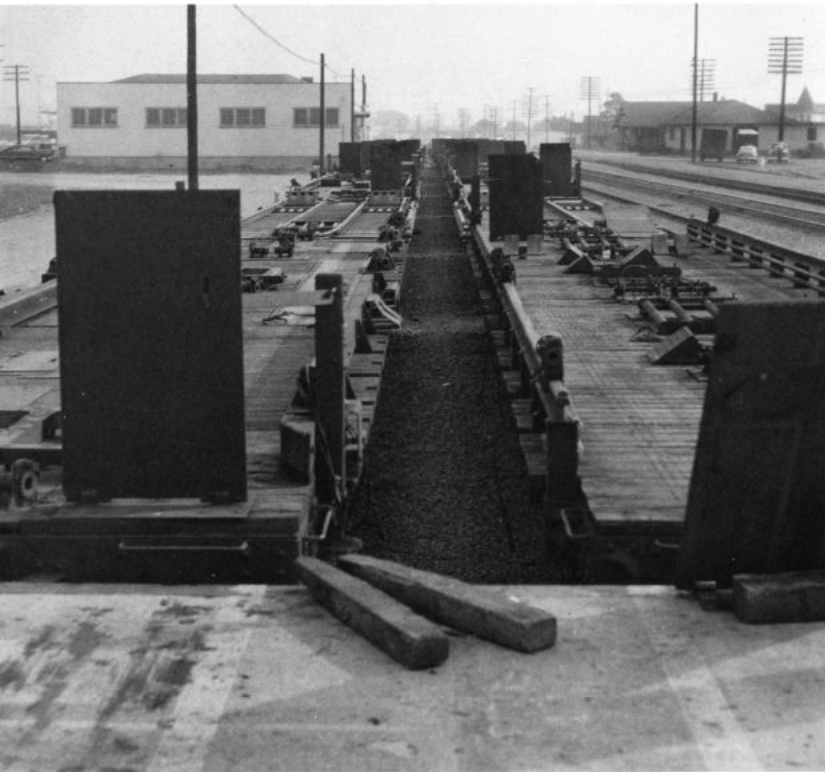
Left and above: This two-track ramp alongside the Cal-P mainlines at Richmond, seen in early 1956, served as the primary Bay Area piggyback staging location until the TOFC complex was completed along Middle Harbor Road in West Oakland in March 1959. —SP photos, John R. Signor collection
