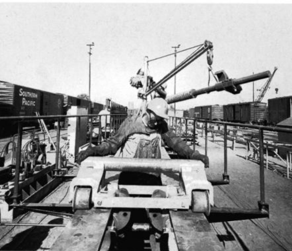
New F-50-17 Class 79-foot 6-inch Clejan-type TOFC cars take shape on the assembly line at Car Shop 9 in Sacramento during early 1957. The open framework of the car can clearly be seen. The clamping device unique to this type of car is seen above. The first of these new cars went into service out of San Francisco in mid-June 1957. —Both Southern Pacific Lines, courtesy Tony Thompson
