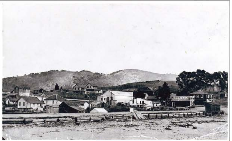
1908 (Continued with) 1910 Retaining wall Poles Anila Water Front
