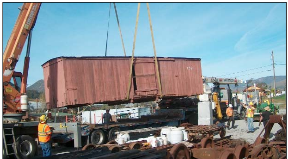
December 19th, Boxcar 706 is lifted off trailer in Emily Street Yard. Full story on page 4
