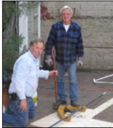
Ted VanKlaveren and Tom Cooper bend and cut new truss rods.
