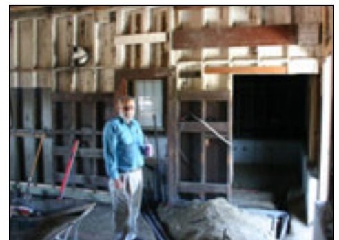
John Marchetti inspects the work on the interior of the Freighthouse.
