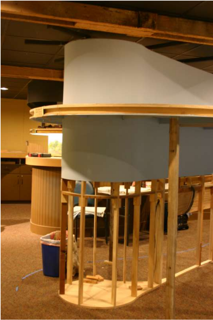
Part of the model railroad benchwork, built by Museum member and skilled carpenter Mike Fairbrother.
