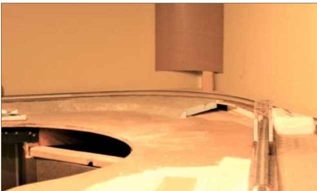
Modelers have installed plywood for the basic horizontal surface and a curved panel for the backdrop.
